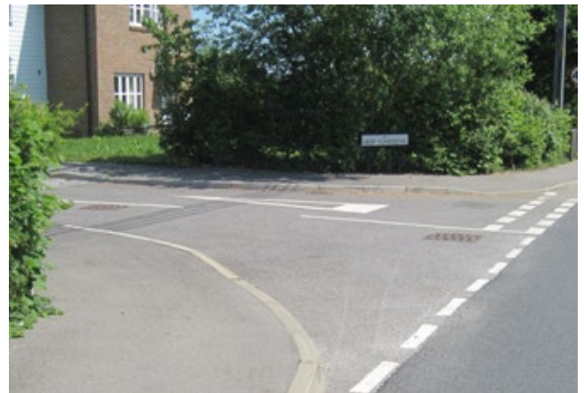
These two road junctions access similar numbers of houses. However, the top image shows a clearly subservient road, reflecting its hierarchy, with tight radii, no white lines, a simple pavement picked out by a small kerb, and traditional materials. In contrast, the image below shows a visually engineering-heavy approach, contrary to MfS and inappropriate for this scale of development in a rural context in the High Weald.
