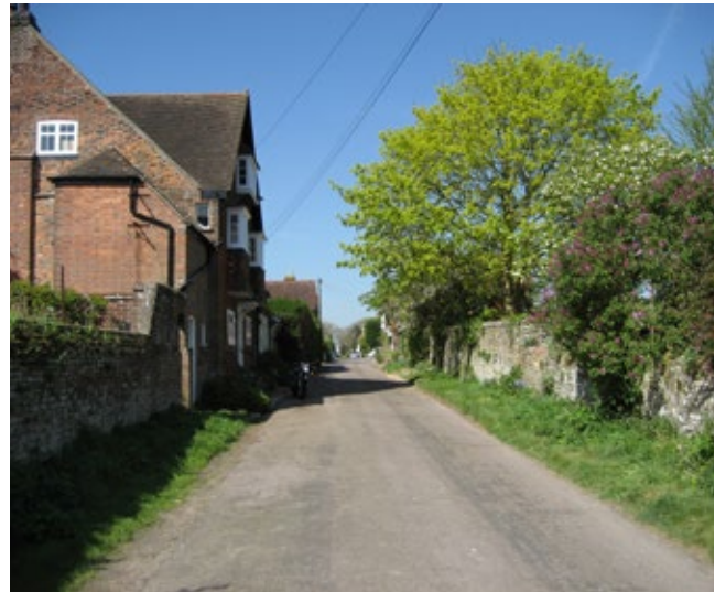
Typical High Weald grass verge detail in residential 'lane'; no pavement or kerb
