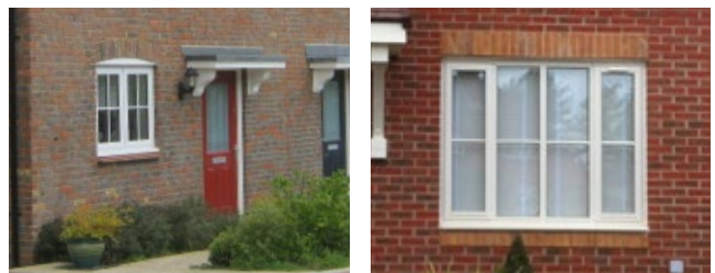
Brick arch over window and inappropriate soldier course
