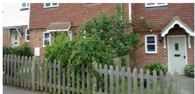
Timber picket fencing to front boundary
