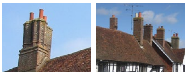
Chimneystacks articulating roofscapes
