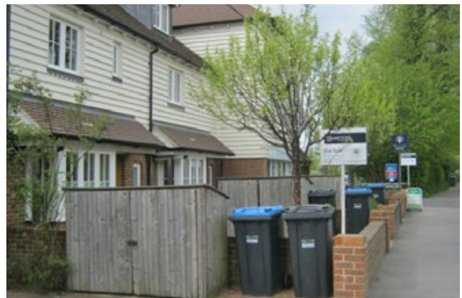
Conversely, the strong building detailing of this scheme is undermined by the forecourt clutter of bins and stores creating a poor streetscene
